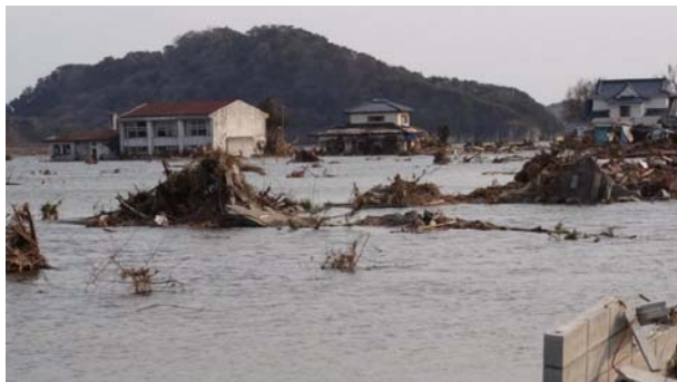
図12 東松島市東名地区の被害. Fig. 12 Damage at Tona area, Higashimatsushima City.
