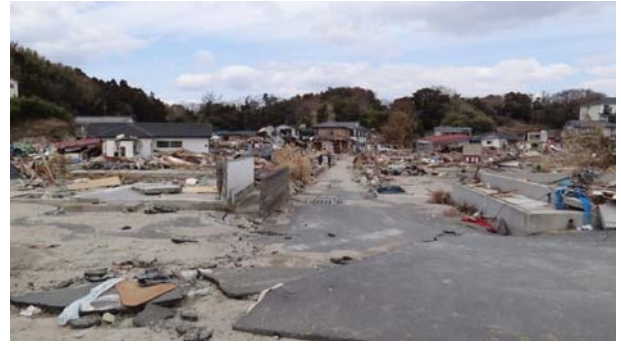
図9 宮戸島月浜地区の被害. Fig. 9 Damage to the houses at Tsukihama, Miyatojima island.
