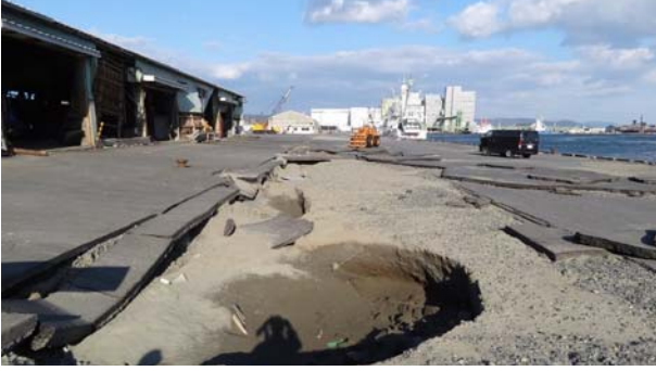
図13 石巻港大手埠頭の被害. Fig. 13 Damage at Oote wharf of Ishinomaki port.
