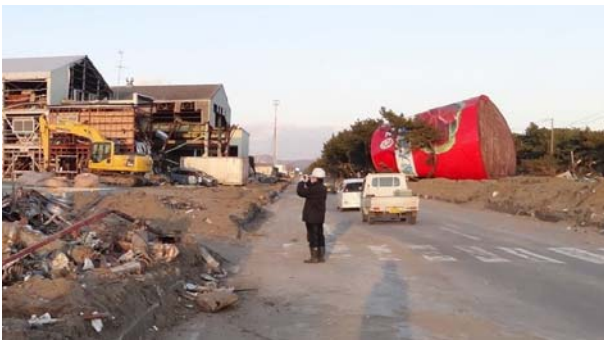
図15 石巻漁港周辺の工場地域の被害. Fig. 15 Damage at the manufacturing quarter near Ishinomaki fishing port.
